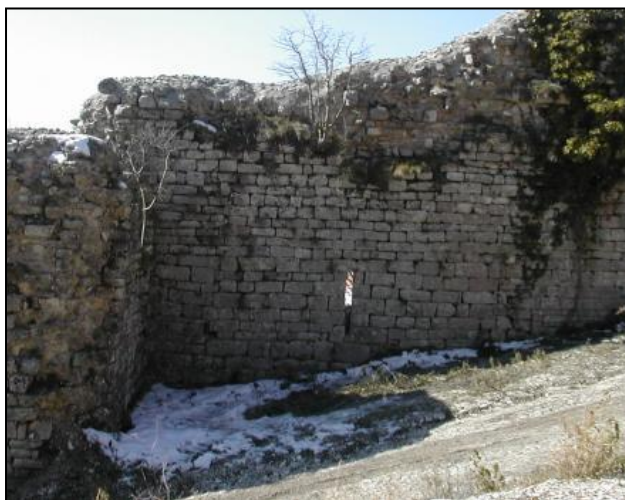
Figure 12 - zone 5: the slope before intervention
