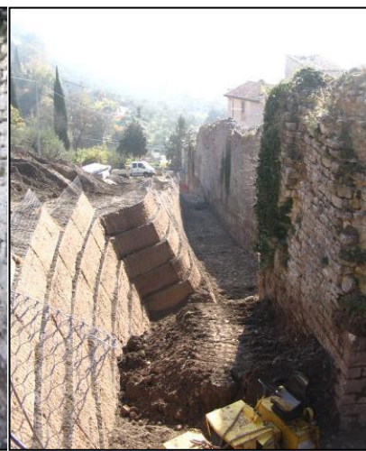
Figure 14 - after excavation during earth-retaining walls building
