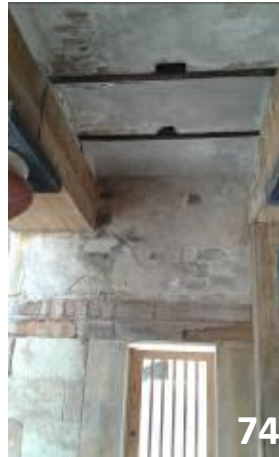
Figures 74 and 75: Light well and Corridor of the "Queen's Megaron". Corrosion of the iron girders used in Evans's reconstruction
