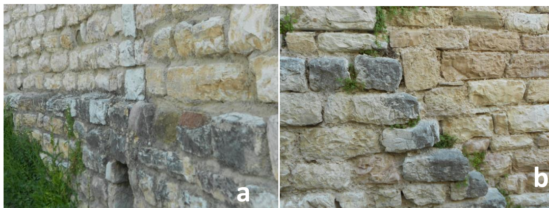
Figure 46 a), b): blackened stone rows on the Walls
