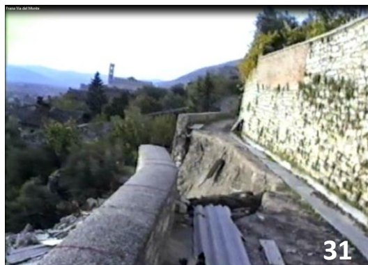
Figures 30-31 - collapse of the medieval terracing under the covering and extending for a greater area with respect to the former problem evidenced by the chasm – just below via del Monte (view from below- east side)
