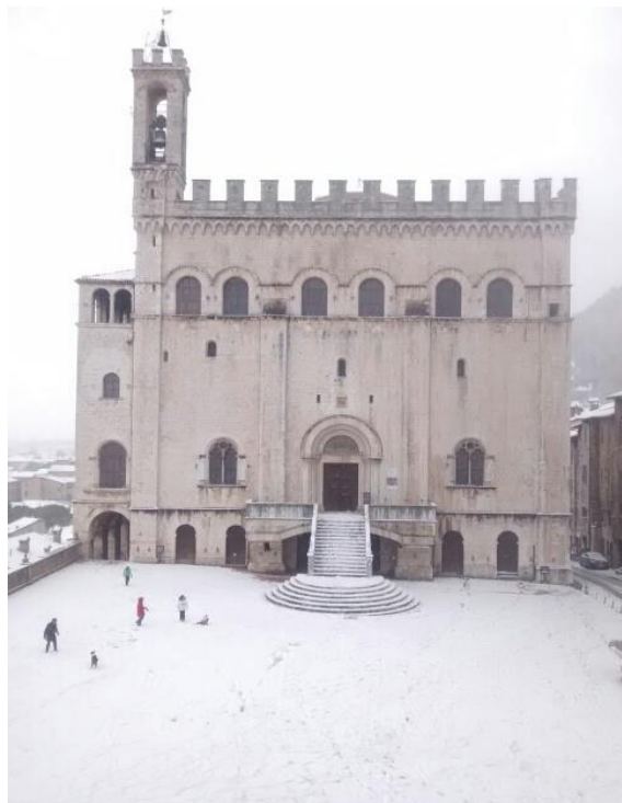
Figure 54- situation of thermal stress and/or freeze-thaw/frost causing damage and deterioration of façades
