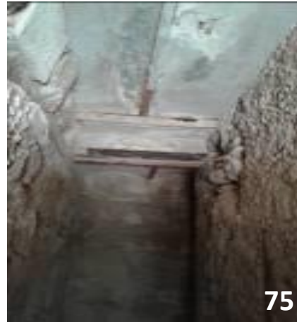
Figures 74 and 75: Light well and Corridor of the "Queen's Megaron". Corrosion of the iron girders used in Evans's reconstruction
