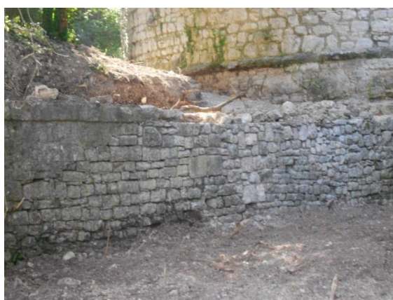
Figure 33- zone 1 - ancient aqueduct retaining wall
