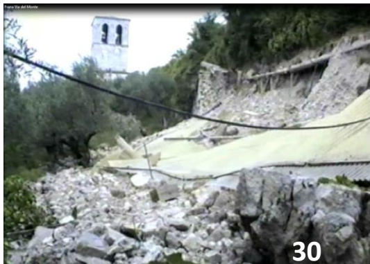
Figures 30-31 - collapse of the medieval terracing under the covering and extending for a greater area with respect to the former problem evidenced by the chasm – just below via del Monte (view from below- east side)
