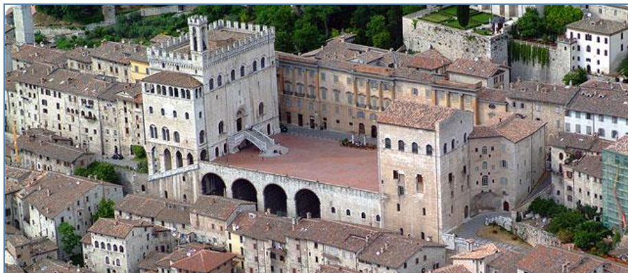
Figure 11: A view of the Consoli Palace complex, in the high part of the town
