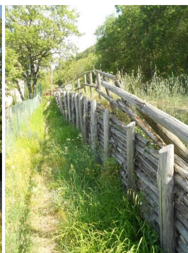
Figure 38- zone 3-4: bended fence
