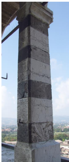
Figure 57 – Consoli Palace-column of the loggia showing differential blackening (limestone).
