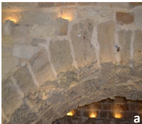
Figures 65 a) and b): Alveolar weathering patterns
