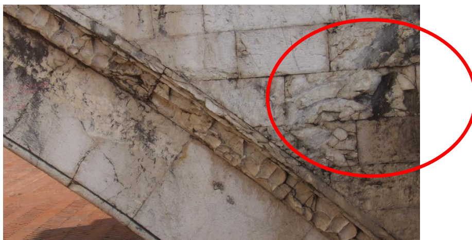
Figure 55 – Consoli Palace- main stairs - freeze-thaw/frost damage causing thermoclasts and consequently loss of material as evidenced inside the red circle.
