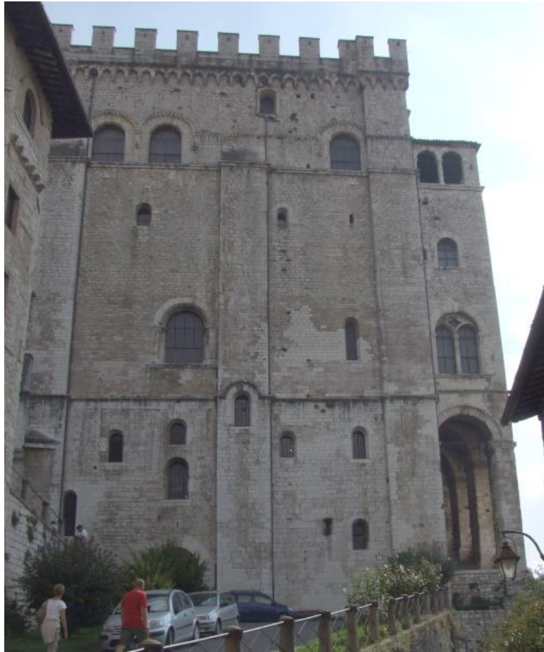
Figure 60- Consoli Palace - black crusts on the façade, view from N-W side
