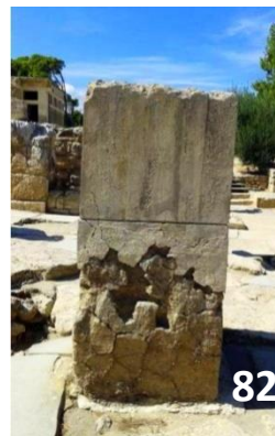
Figures 81, 82: Crack & Deformation; Secondary mineral gypsum from the “King’s Megaron” showing a network of thin cracks. Cracks due to mechanical stress from the “North Entrance”.
