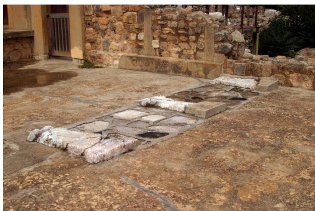
Figure 88. Eroded (dissolved) gypsum slabs from the “King’s Megaron”, Palace of Knossos.
