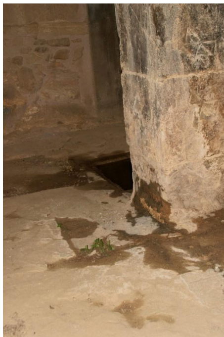
Figure 92. Salt efflorescence, growth of higher plantation and rain water accumulation (after the rainfall on the 31 st of October 2016), "Pillar Crypts", Palace of Knossos.
