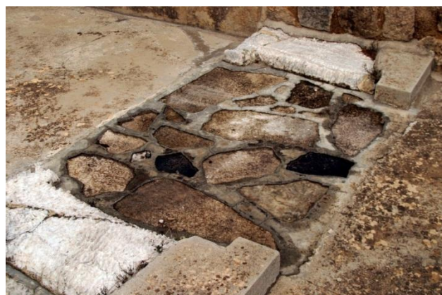
Figure 89. The dissolved gypsum elements are preserved in a lower level comparing to the cement mortar that was initially used for the fixation of the gypsum fragments, “King’s Megaron”, Palace of Knossos.
