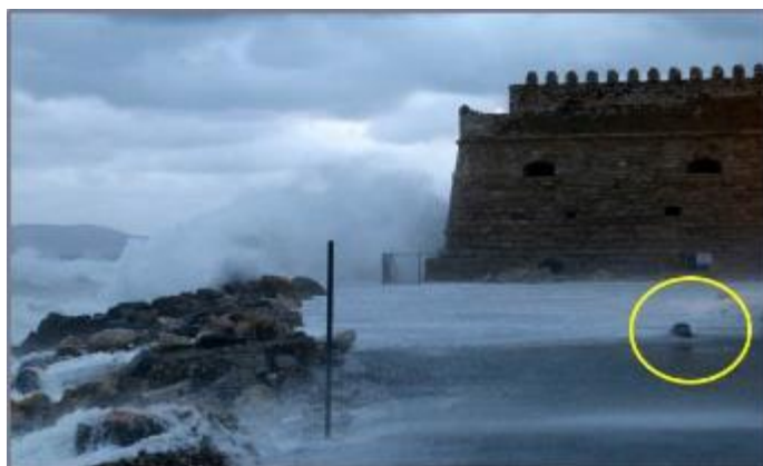
Figure 69: Example of structural risks due to the impact of big pieces of rock (highlighted in the yellow circle) from the breakwater structures upon intense wave events
