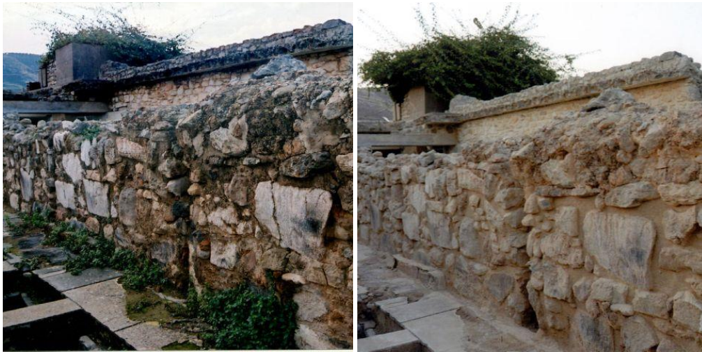
Figure 6: Minoan walls before and after the conservation works.
