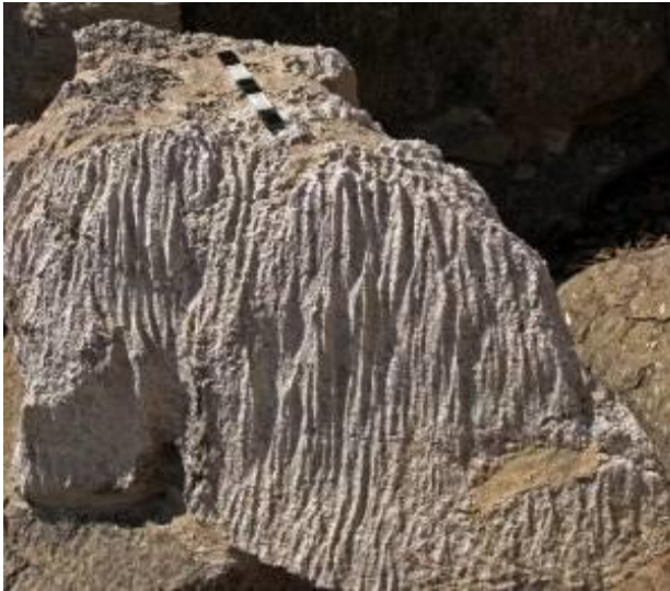
Figure 20: Microkarst runnels on the surface of a building element located near the west magazines, Palace of Knossos.
