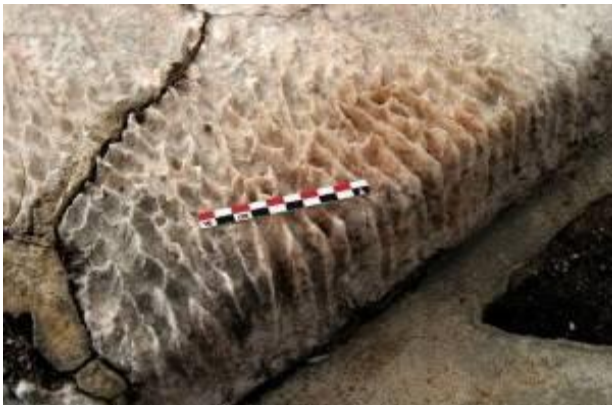
Figure 19: Typical formation of microkarst cavities on the surface of secondary gypsum from Knossos. Dissolution pits, grooves and runnels, collectively called karren.
