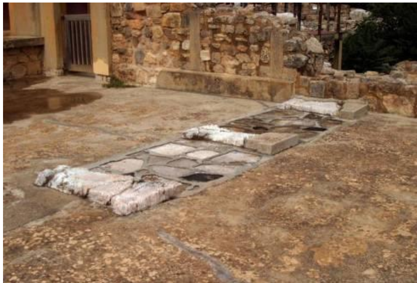
Figure 25: Eroded (dissolved) gypsum slabs from the “King’s Megaron”, Palace of Knossos.
