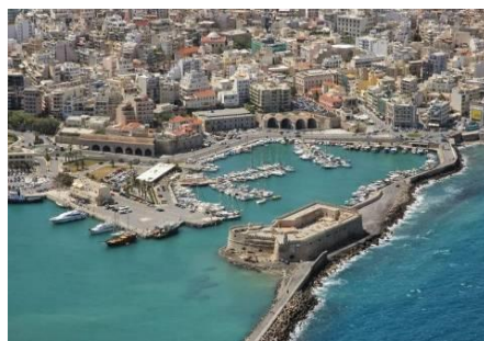
Figure 46: Aerial photo of Heraklion port and Koules fortress.
