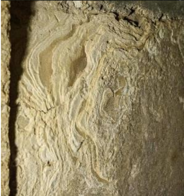
Figure 16: Exfoliation of microcrystalline mineral gypsum slab, Palace of Knossos.
