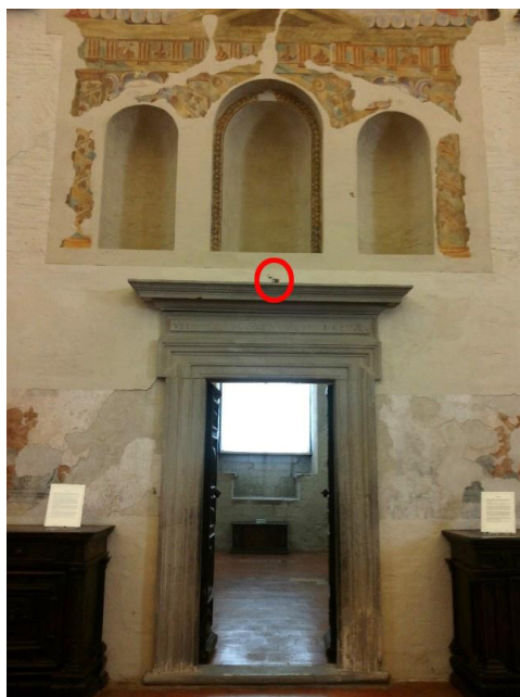
Figure 28 - Thermo-hygrometer location within the Consoli Palace
