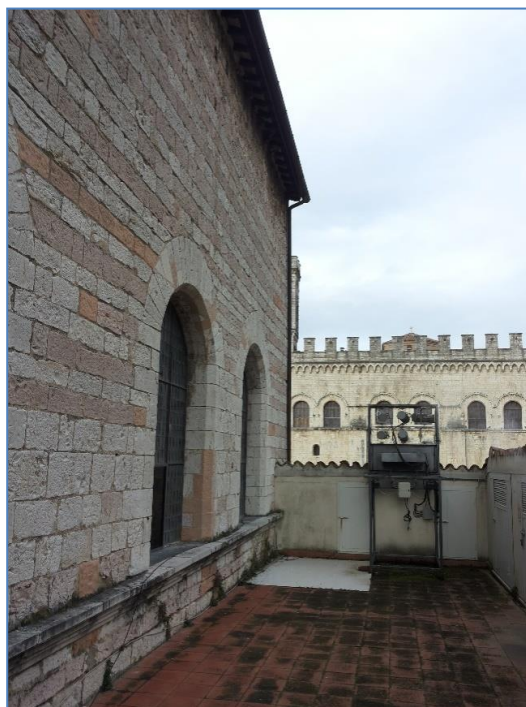
Figure 30 - Gubbio municipality building terrace where the sensor is located
