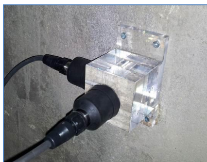
Figure 33 - Accelerometers used for the dynamic monitoring of Consoli Palace.
