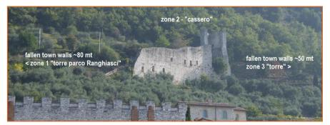
Nowadays, climate change is a threat for the preservation of the Walls. They mainly suffer from heavyl rains and humidity characterizing the soil surrounding the area, closely connected with the mountain natural zone. The heavy rains increase the push on the Walls in two ways: the first one is through the washout
